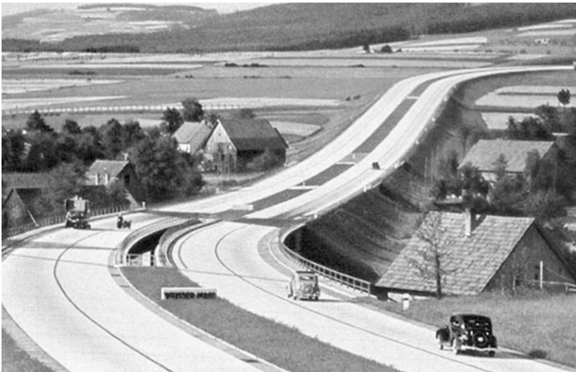
By September 1939 the Reichsautobahn covered 2,400 miles (3,862 km). It was aesthetically designed to serve not only a utilitarian purpose, but to provide the motorist with scenery and
